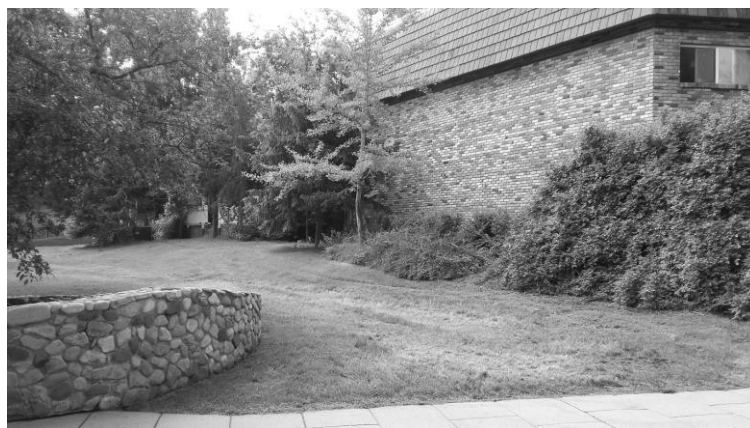
Figure 2- Photograph of the proposed relocation site showing no windows on the South facing wall of the Victoria House Apartments.
